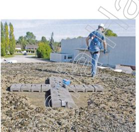
The **Blocfor™10** AES is Personal Protective Equipment (PPE) compliant with the requirements of standard EN 360 and the utilisation requirements for work conducted on terraces as defined by the technical data sheet of VG11 dated 2009. To meet these requirements, the fall arrester must be equipped, optionally, with a two-meter strap lanyard (code 035032).
