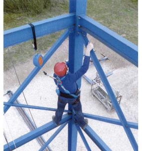
The **Blocfor** 10 AES, automatic fall arrester is equipped with the new AES system (**Absorbing End System**) patented by **Tractel**. The AES system ensures that the user will be exposed to an impact of less than 600 daN even if he falls with the wire rope fully unwound. The AES system reduces the violence of the impact on the user's body and protects the end of the lanyard against the risks of breaks due to sharp edges on terrace roofs.
