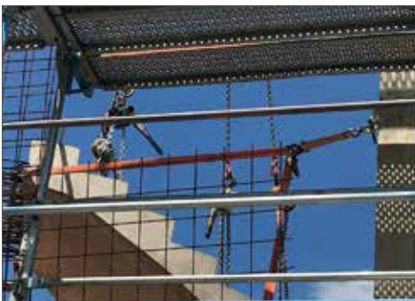
Positioning of loads Especially when using multi-fall chain slings (e.g. installation of stair segments and turbines)
