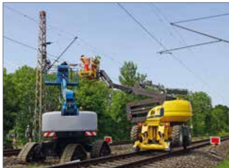
Construction of contact lines
